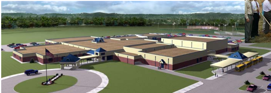
South Claiborne County High School, Tazewell, TN
