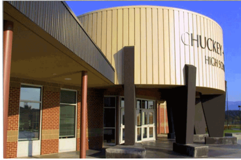
Entry of Chuckey-Doak High School in Greene County, opened in the Fall of 2004 for $94 per square foot.
